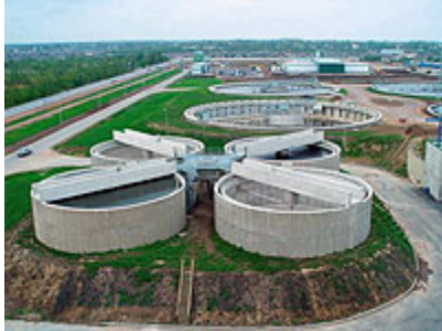
Approximately 2,000 kg of KIM-HS was used in the St. Petersburg Southwest Wastewater Treatment Plan.
