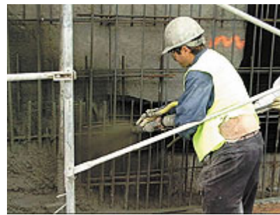
ACI-certified nozzleman applying shotcrete with KIM®
