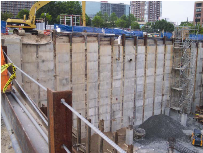
Krystol waterproofing technology eliminates the need to access the exterior surface of the structure.
